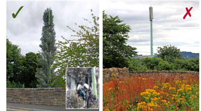
Good example of disguised equipment
