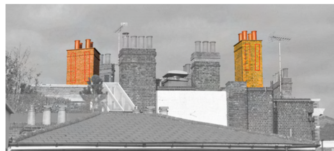
Good example of equipment disguised within existing structures Photographs courtesy of Dynamic Concepts
