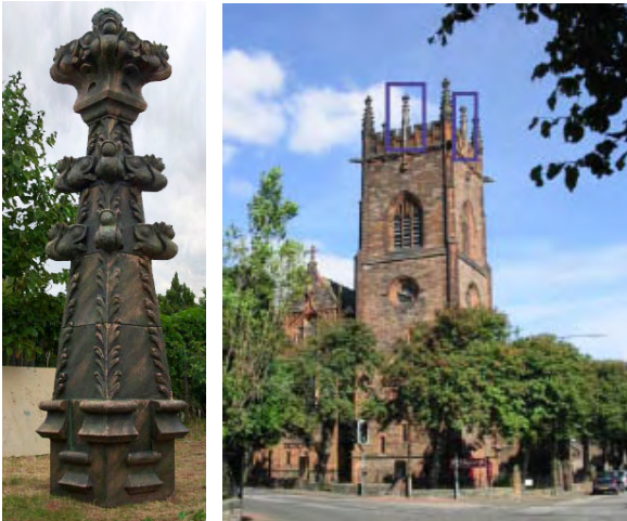
A silicon mould was taken from the original pinnacle
